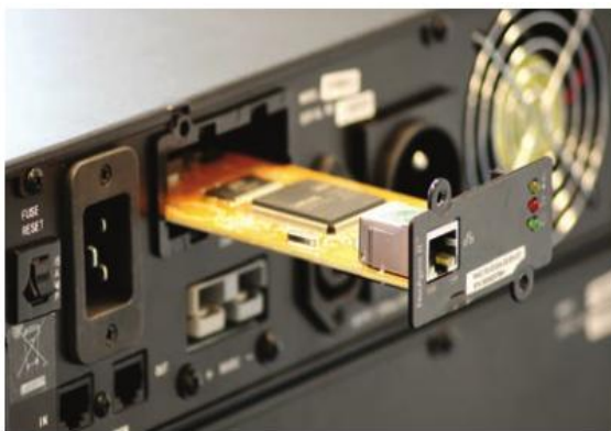
Installation of an internal SNMP card into rack-mount SJ900 UPS
